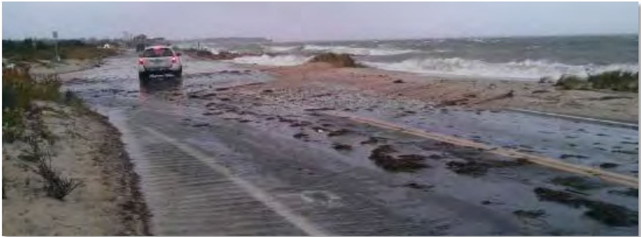
Figure 3-3. Flooding on Surf Drive during Hurricane Sandy.
