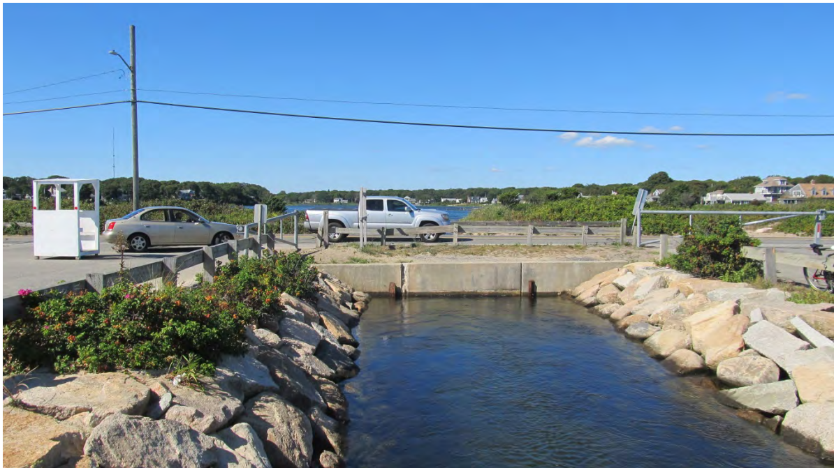
Figure 3-29. Culvert at Little Pond inlet.
