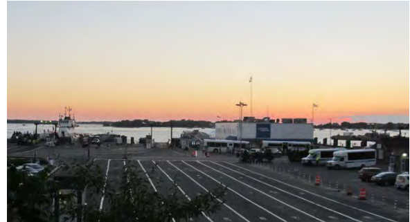
Figure 4-5. Steamship Authority Ferry Terminal
