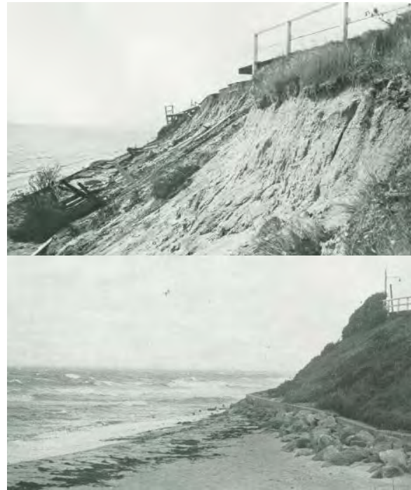
Figure 3-6. The coastal bank fronting Grand Ave. at Falmouth heights immediately after the Hurricane of 1938 (top) and following restabilization (bottom).
