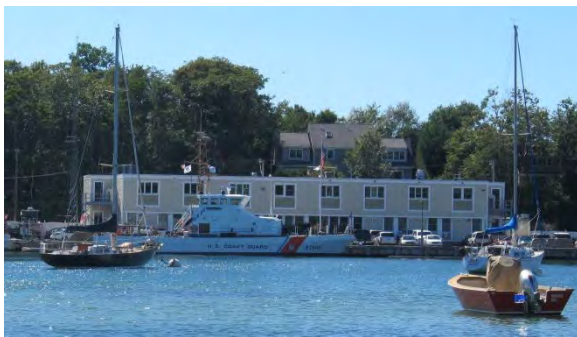
Figure 4-4. Woods Hole Coast Guard Station
