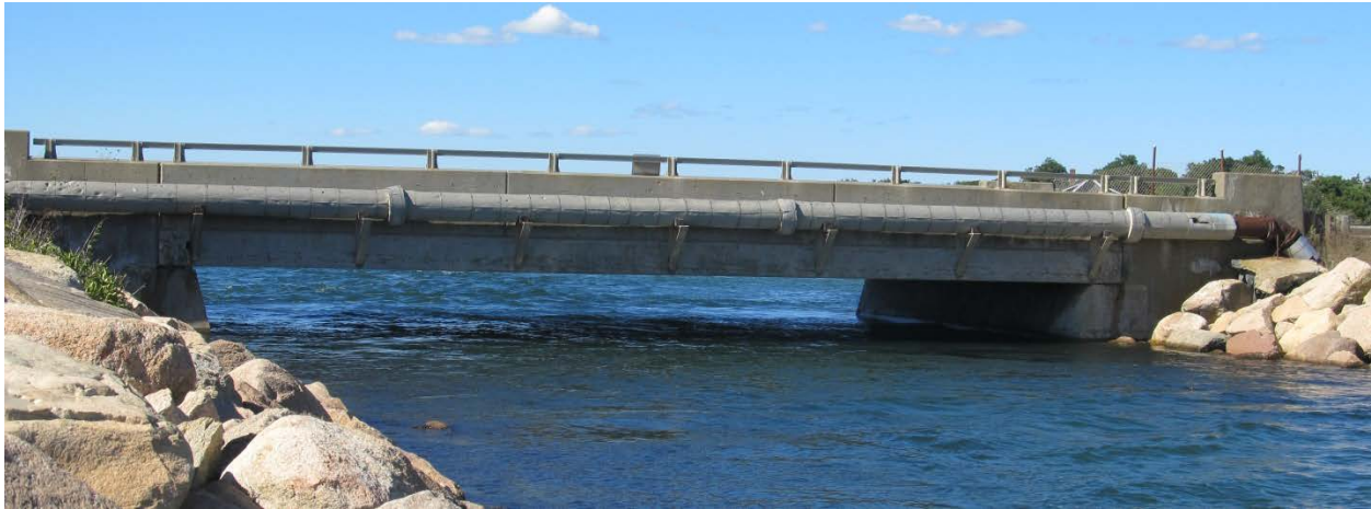
Figure 2-9. Water main on Bourne's Pond Bridge.
