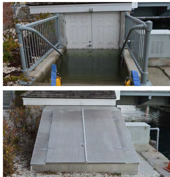
Figure 4-3. Woods Hole Drawbridge Hut flooded immediately after Tropical Storm Sandy (top) and after bulkhead construction (bottom).
