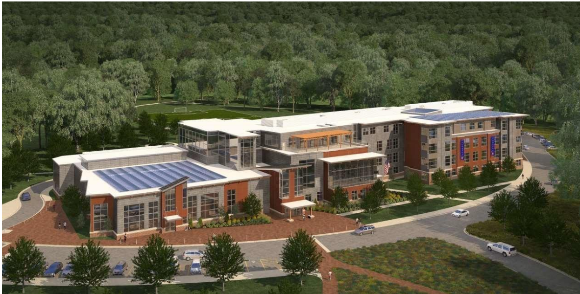
PHOTO ABOVE: RENDERING OF NEW KENNEDY MIDDLE SCHOOL. THE SCHOOL WILL FEATURE A 403 kW AC SOLAR PV CANOPY AND ROOFTOP SYSTEM AND A 223 kW AC BATTERY STORAGE SYSTEM. COMBINED THE SYSTEMS ARE EXPECTED TO SAVE NATICK PUBLIC SCHOOLS $1.7 MILLION ON ENERGY COSTS OVER THEIR 20 YEAR LIFE.
