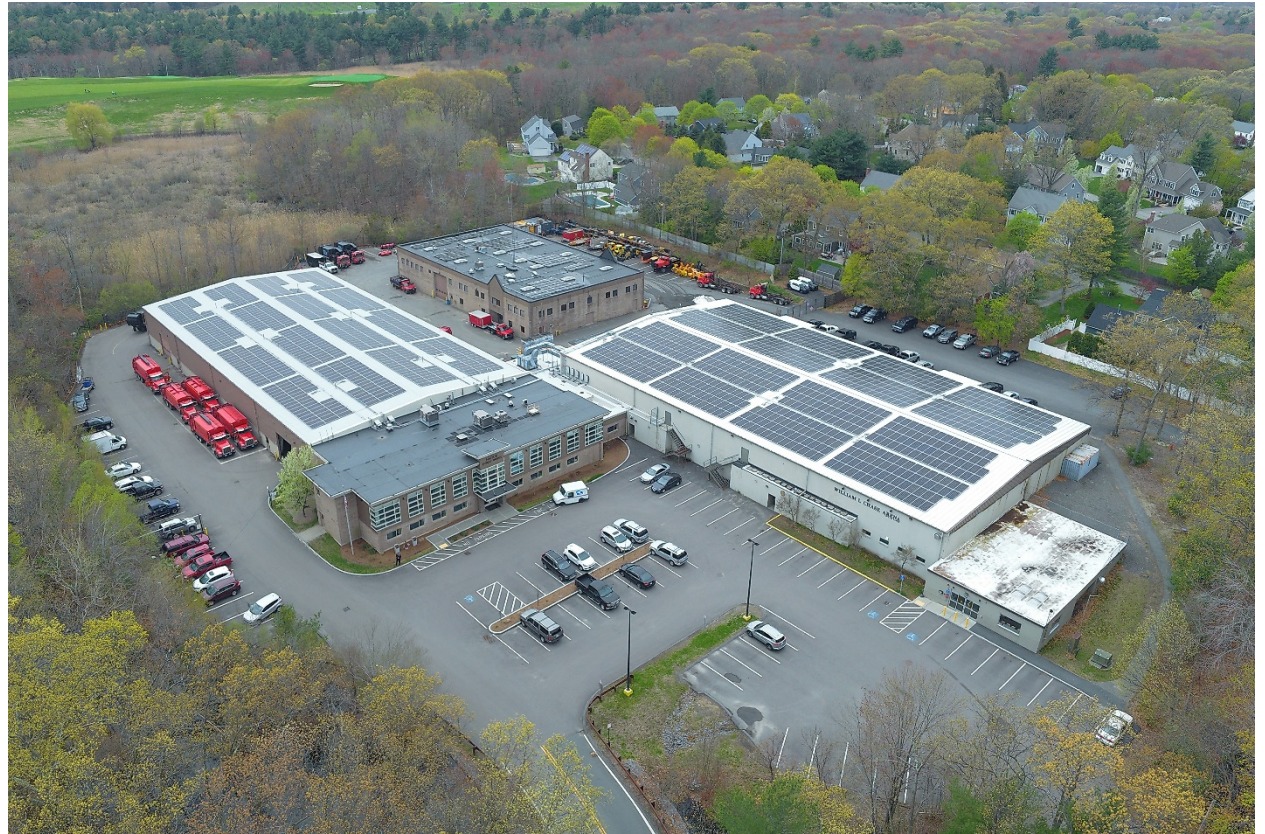
PHOTO ABOVE: SOLAR INSTALLATION AT NATICK'S DEPARTMENT OF PUBLIC WORKS BUILDING
